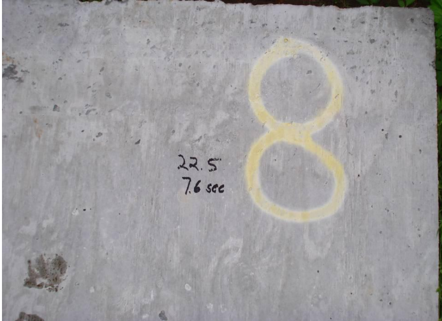
Figure 2: A close-up example of a wall section
