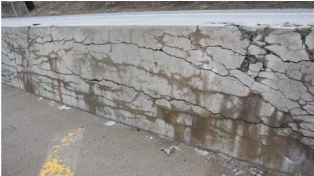
Figure 2. Barrier wall exhibiting ASR deterioration.
