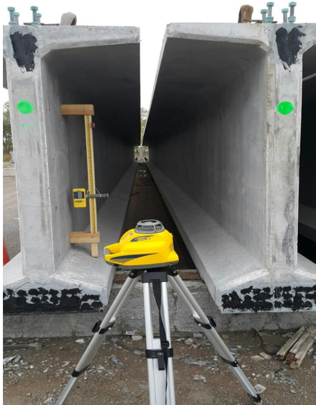
Figure 3. Rotary Laser Level with Receiver Used in Camber Measurements
