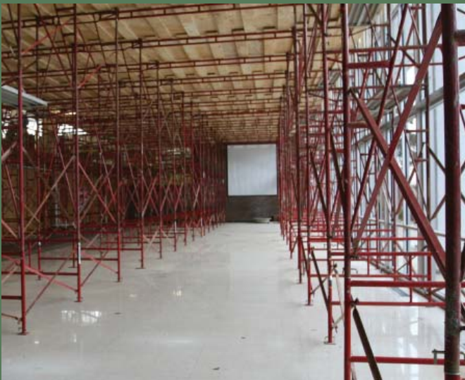
Asbestos Abatement at Pomfret Great Room
