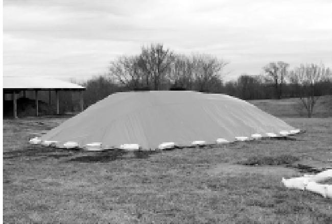
Figure 1. Free-standing wind-row litter storage system with tarp cover. Pile cross-section has dimensions 20 ft. bottom width, 3 ft. top width and 6 ft height. Tarp is 30 ft. wide, 6 mil thick, 3-ply polyethylene. Sandbags placed every 2 to 3 foot along the perimeter hold the tarp down.
