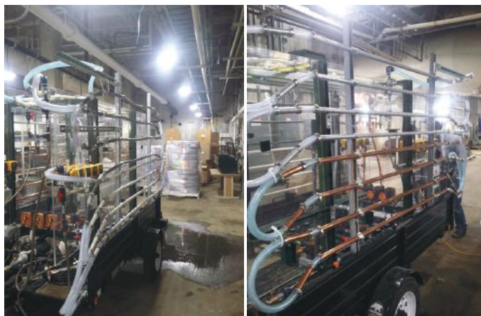
Figure 2 (left) and 3 (right). On the left, a pipe loop displaying PEX-A train (on top of pipe loop), Galvanized Steel train (top of loop wall) and Copper-K train (bottom of loop wall). On the right, a pipe loop displaying Lead train (top of pipe wall) and PVC train (bottom of pipe wall).
