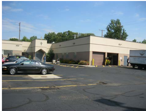
Figure 4.19 Earthworks Restrooms in Soup Kitchen
