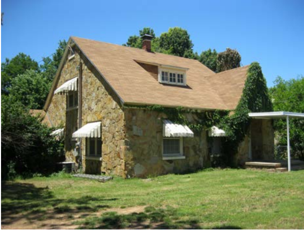
Figure 4.16 Tricycle Farm restrooms in Building
