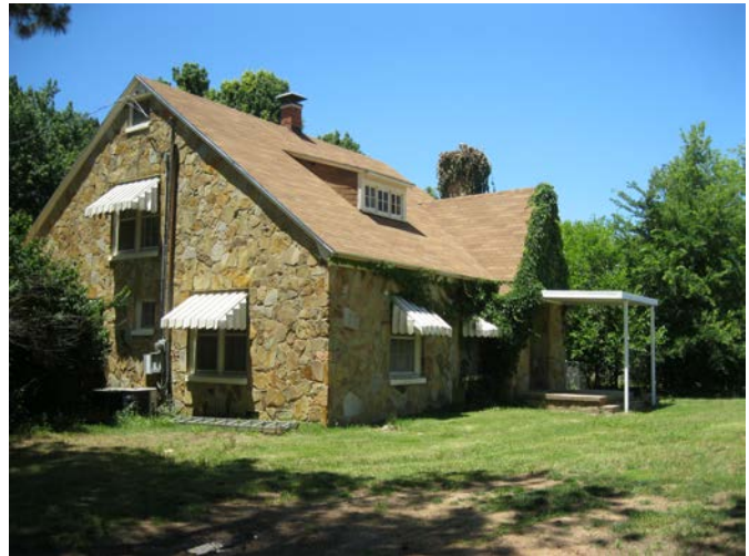
Figure 3.8: 1920s House as Office , Photo by D. Freeman 8/14
