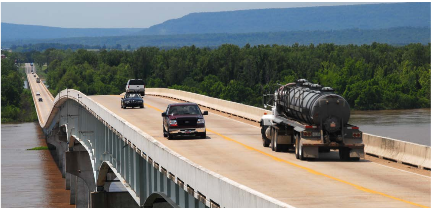
Clarksville Bridge, Highway 109 - Photo courtesy of AHTD
