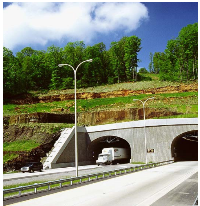
I-540, Bobby Hopper Tunnel - Photo courtesy of AHTD
