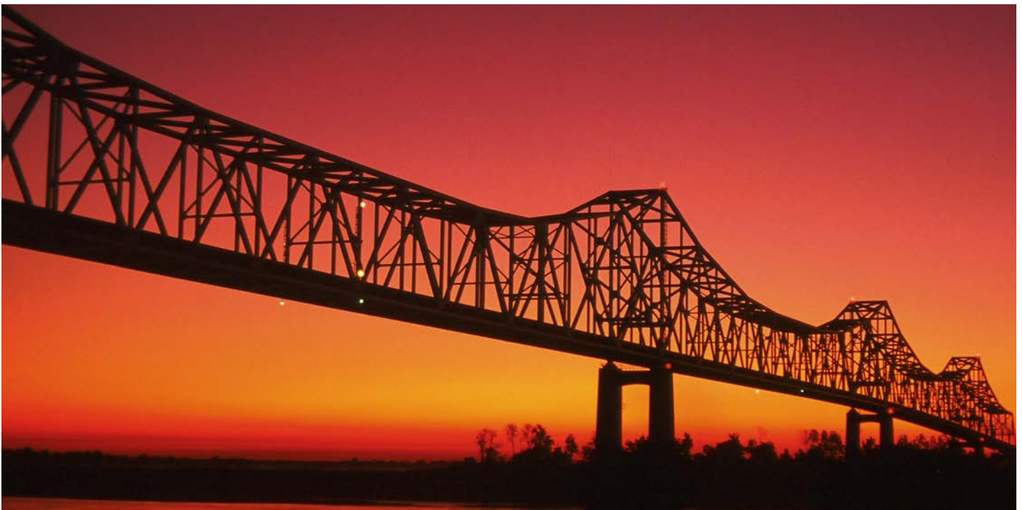
Helena Bridge, Highway 149 - Photo courtesy of AHTD
