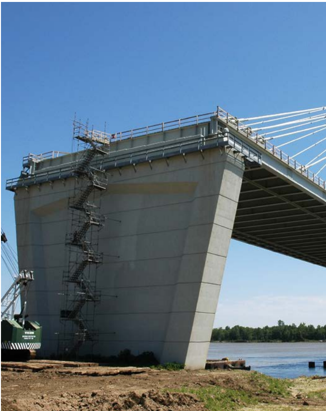
Greenville Bridge Construction - Photo courtesy of AHTD
