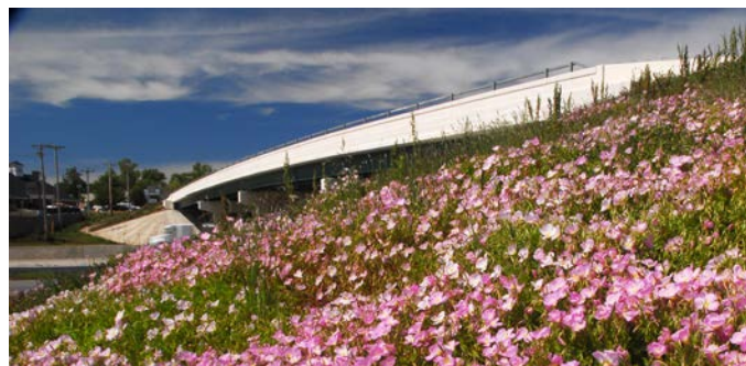
I-30, Saline County, Exit 117 - Photo courtesy of AHTD
