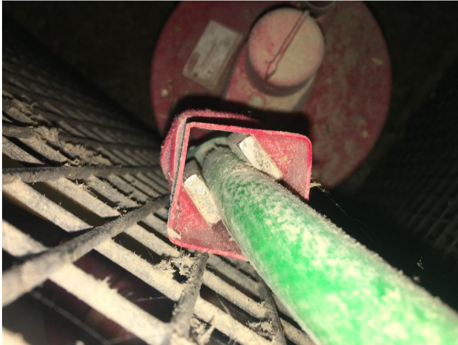
Image 2: Attachment of small N52 Neodymium magnet used to magnetize water for treatment 3
