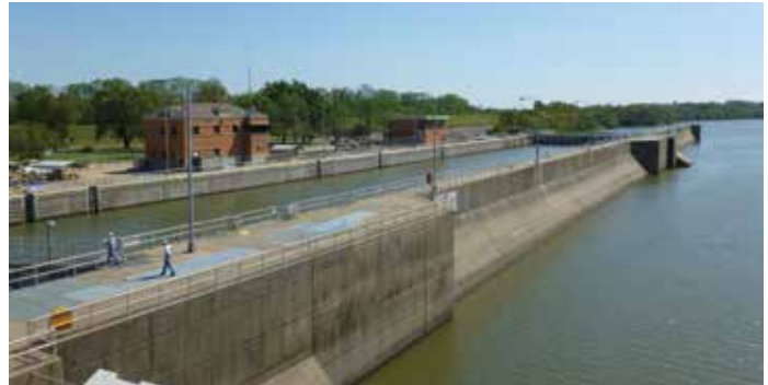
Newt Graham Lock and Dam (L&D #18) near Tulsa, OK
