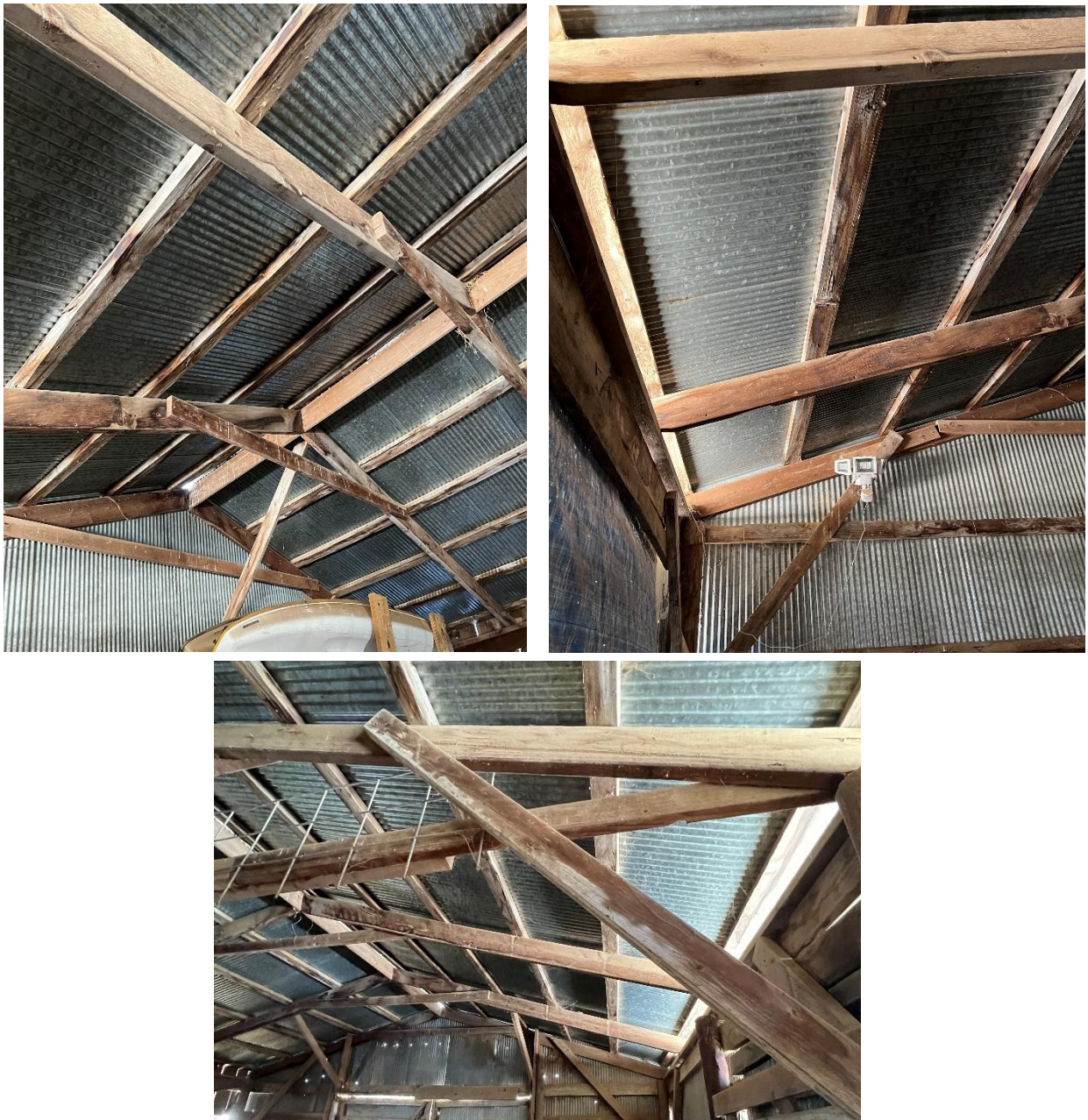
Example of roof support beams:
