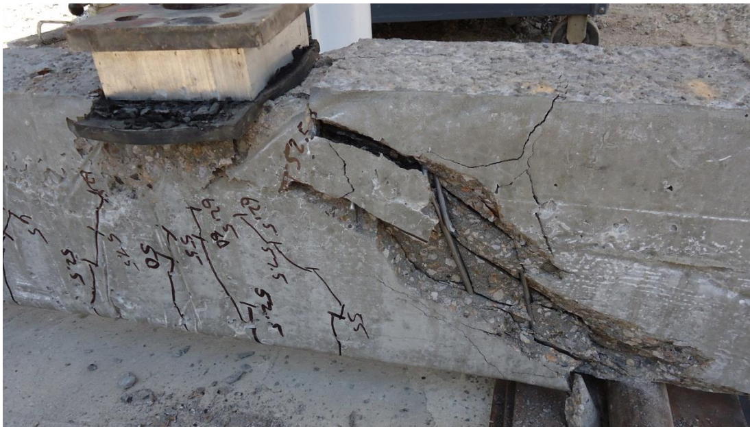
Figure 3. Clay 4 Dead End Test – Typical Web-Shear Failure
