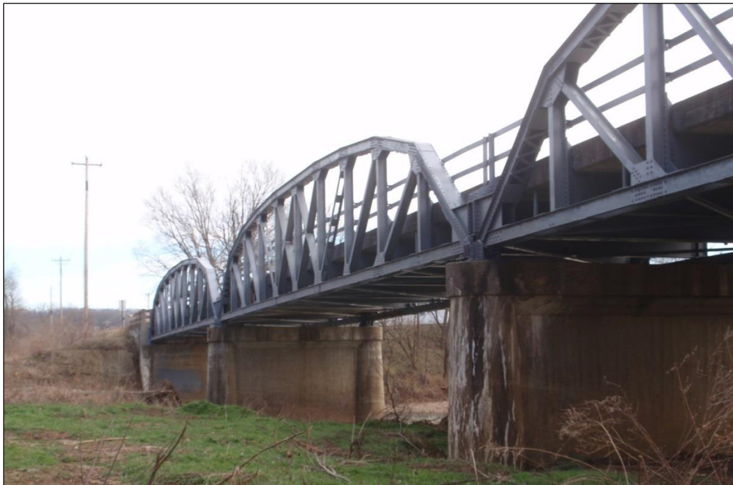
Figure 2. Photograph of the truss bridge that was tested.
