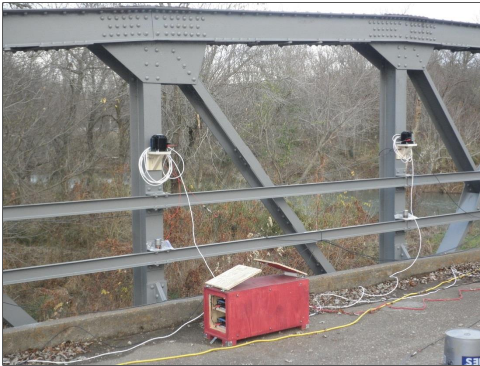
Figure 4. Experimental equipment installed on the bridge during vibration testing.
