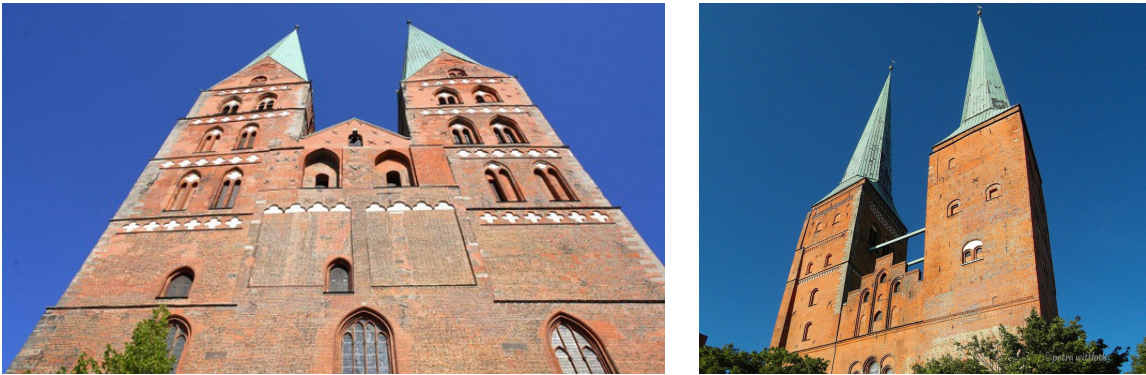
Figure 36. Comparing the Gothic towers of Lübeck's Marienkirche and Dom
