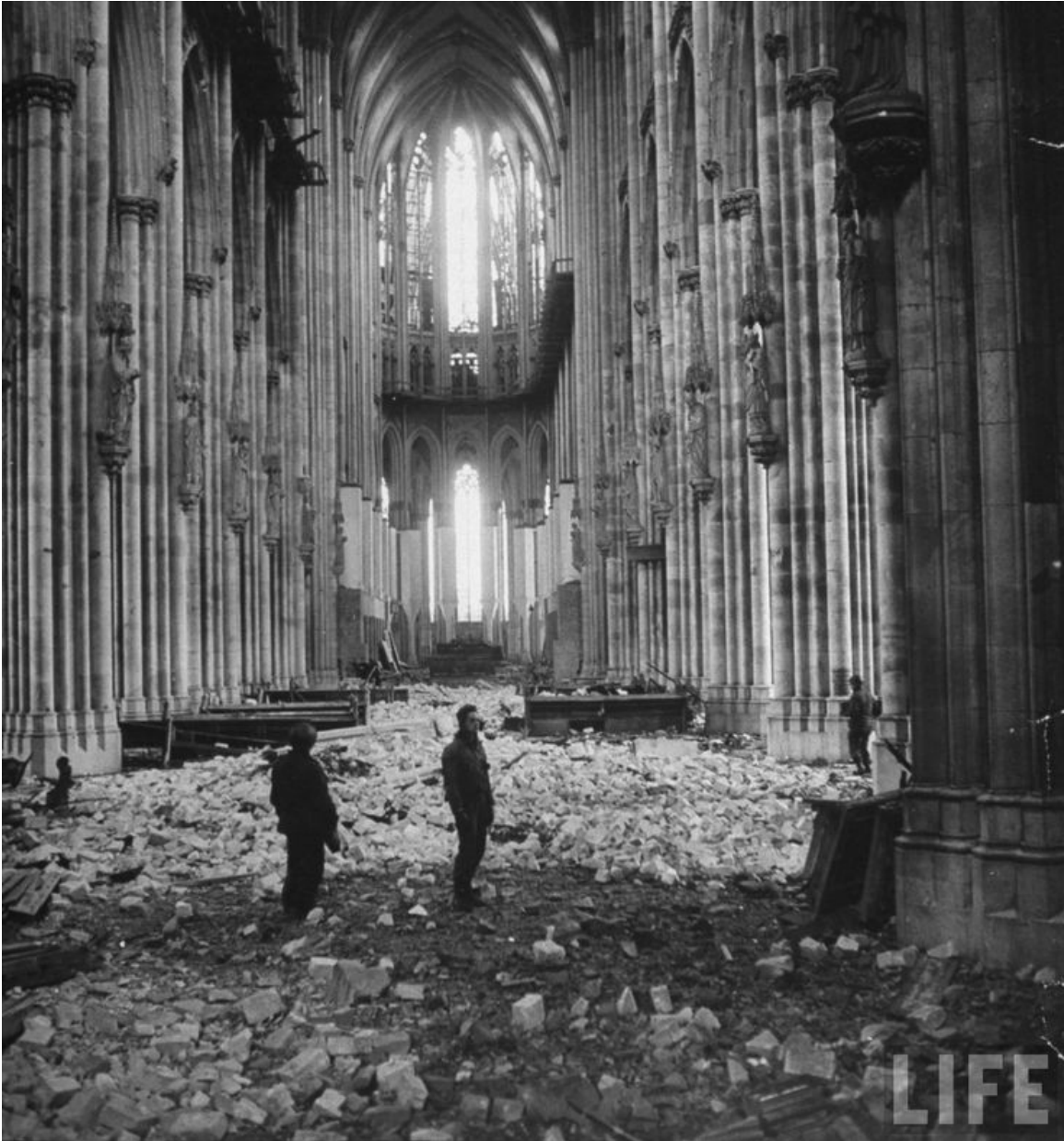
Figure 23. Rubble in Cologne Cathedral, 1945
