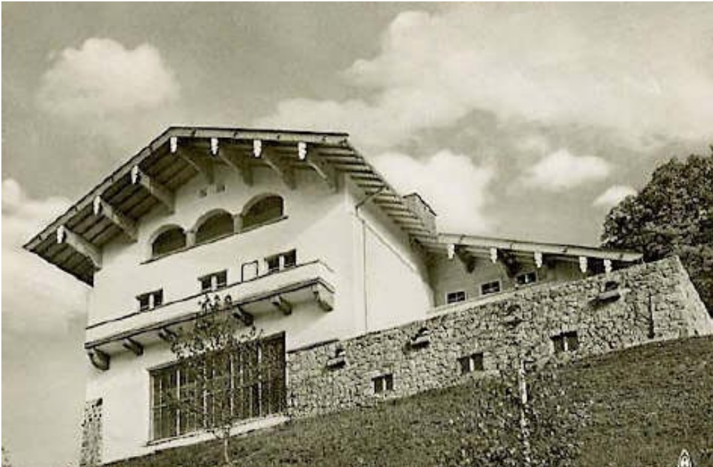
Figure 5. Hitler's personal residence, "The Berghof," Obersalzberg, 1933-35, demolished 1952
