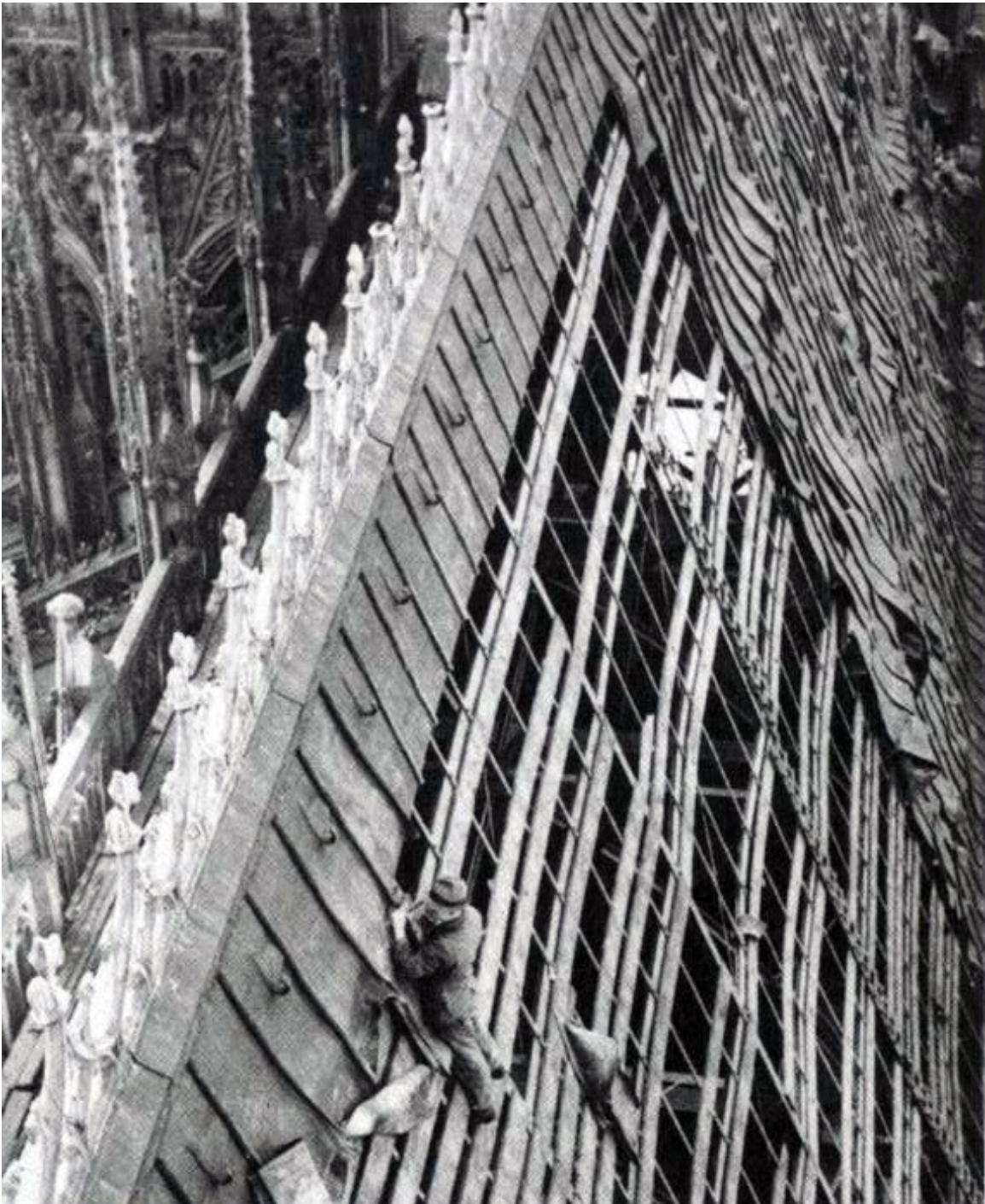
Figure 24. Roof panel reconstruction at Cologne Cathedral
