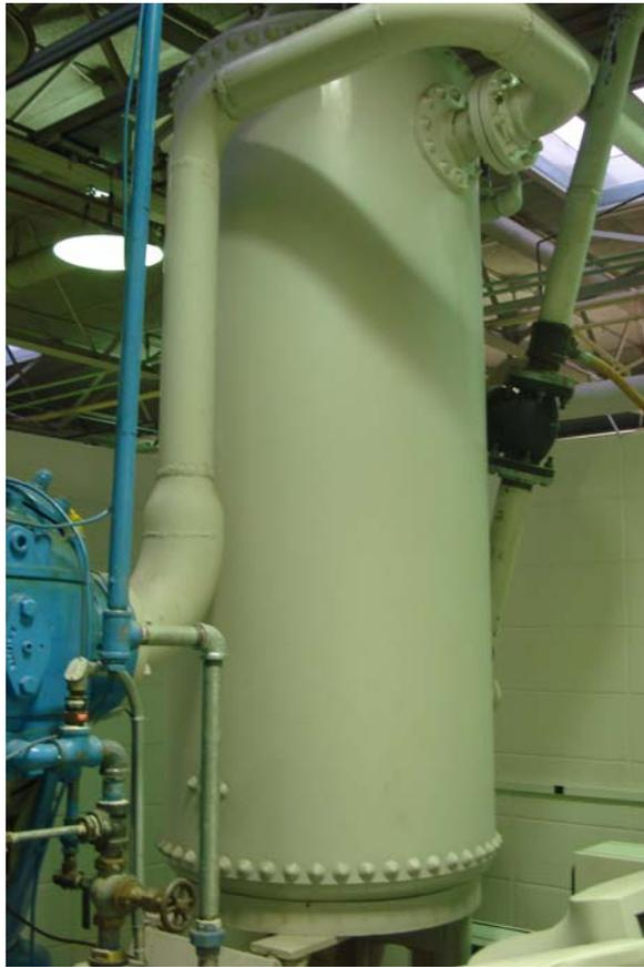
**Figure 1:** The existing compressed air tank at the Mechanical Engineering building at the University of Arkansas
