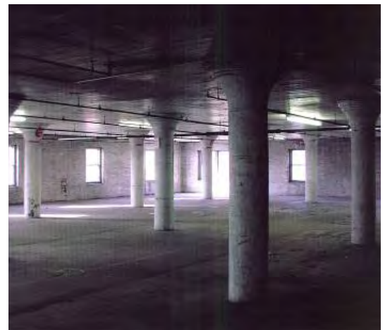
Patent for "Mushroom Columns" and the Green & DeLaitre Wholesale Grocery Company Warehouse, Minneapolis
