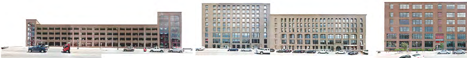
Fig. 32 - Washington Avenue Street Front
