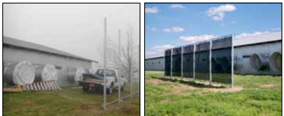
Figure 3. Structural windbreak wall installation on the broiler farm
