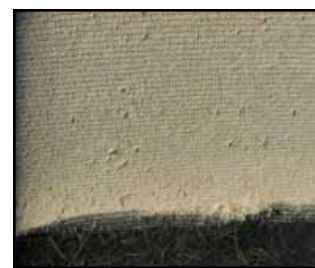
Figure 7. Windbreak walls are effective in trapping dust and feather blown by the tunnel fans out of the chicken house
