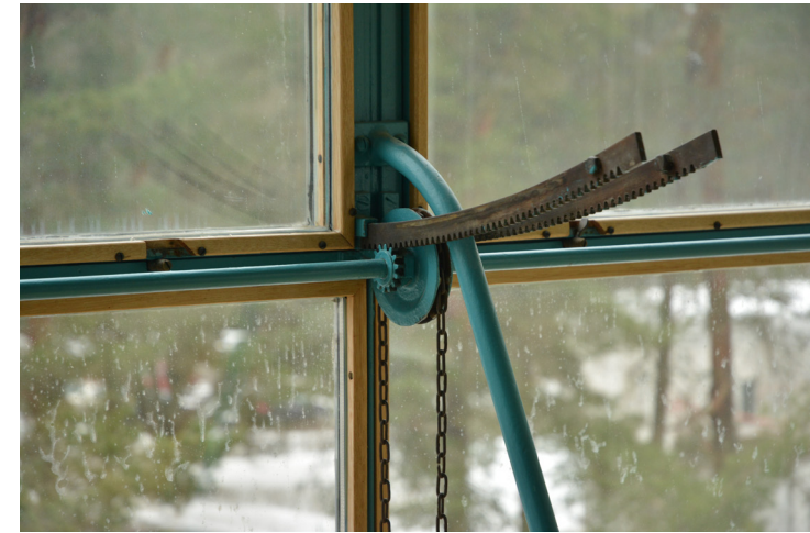
Alvar Aalto. Sannitorium. Window detail. Easily Operable window brings outside in.
