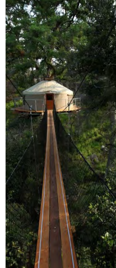
The Lofthaven is a single tree layout treehouse, the hardest to complete. The hoisting of beams, drilling of trees, and creation of the platform is a tall order in a single tree layout.
