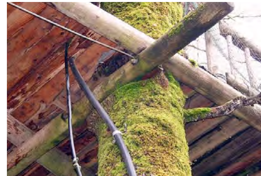
Illustrated need for a better fastener- tree grows into treehouse supports
