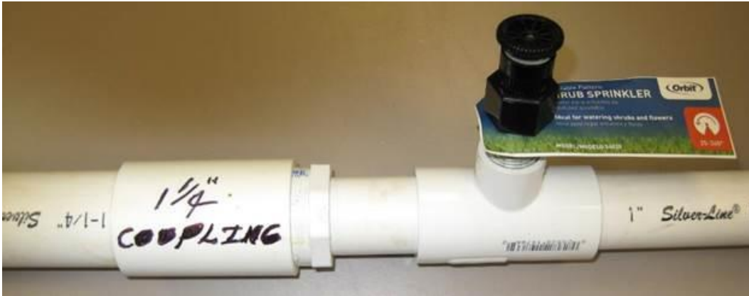
Figure 7. Decreasing pipe diameter from 1.25" to 1" with sprayer.
