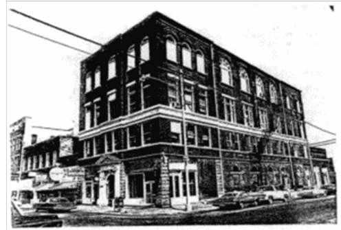
Figure 5. Grand Masonic Temple Exterior
