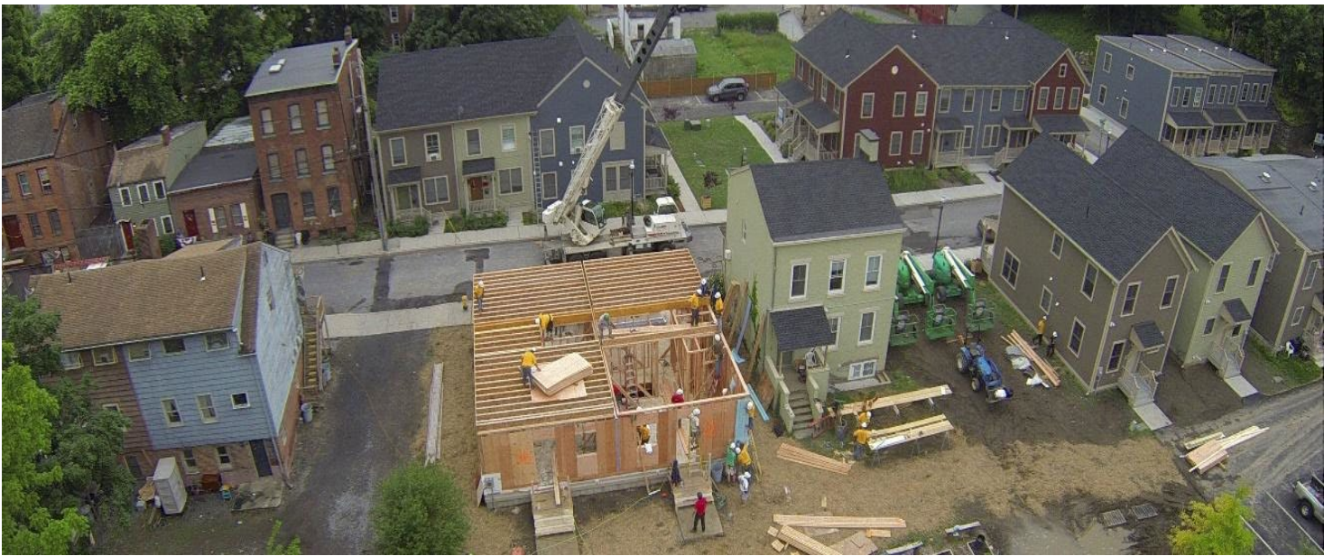
Figure 27, Habitat For Humanity's project in construction
