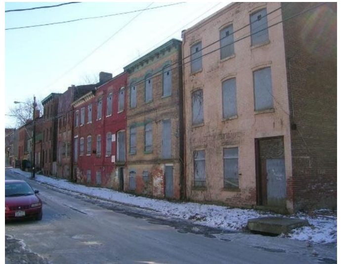
Figure 25. Poor Quality Housing in Newburgh
