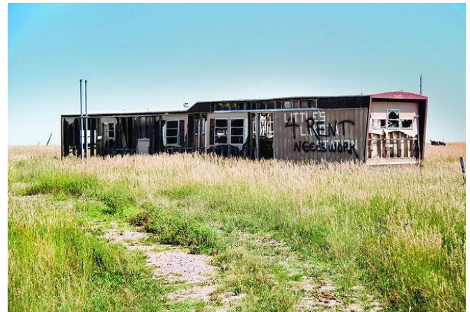
Figure 14. Poor Quality Housing in Pine Ridge
