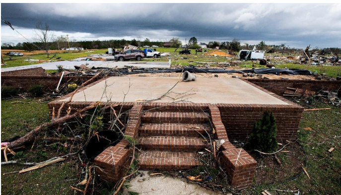
Figure 2. Tornado Aftermath in Dallas County
