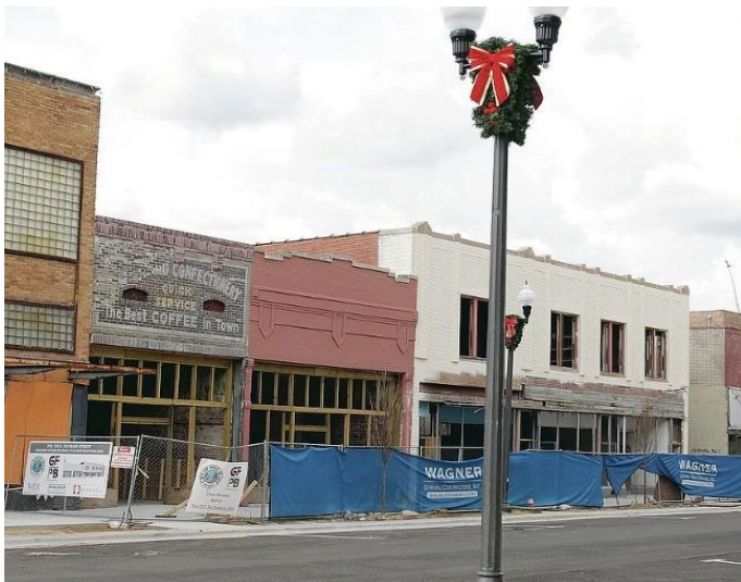
Figure 4. Abandoned buildings in Pine Bluff
