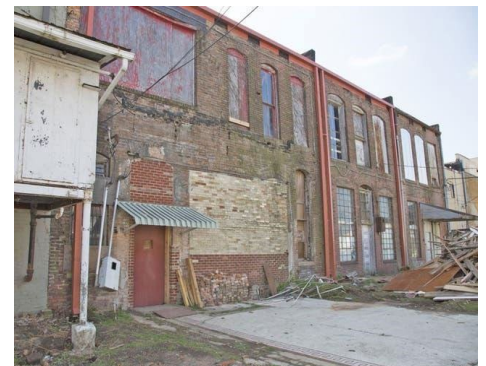
Figure 2. Abandoned buildings in Pine Bluff
