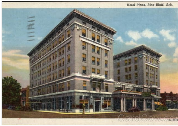
Figure 9. Hotel Pines Exterior
