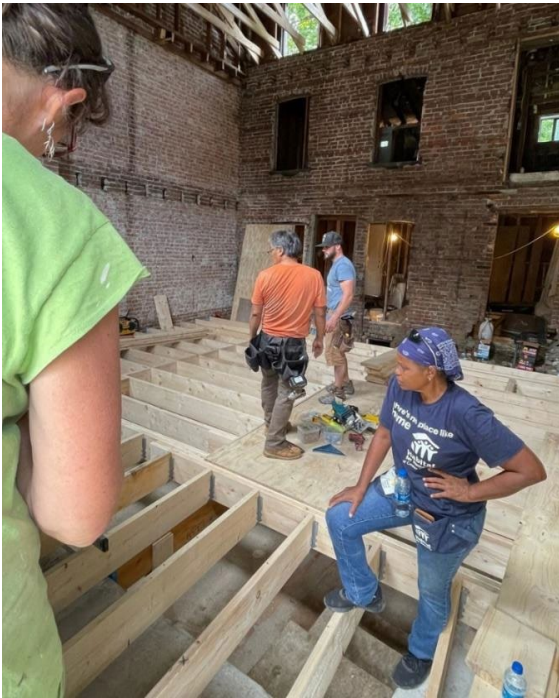
Figure 30. Habitat for Humanity's Home in Construction
