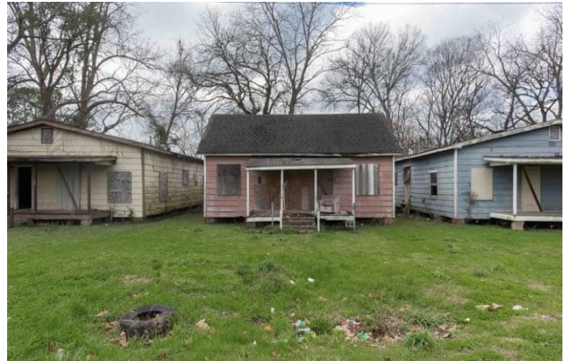
Figure 3. Poor Quality Housing in Dallas County
