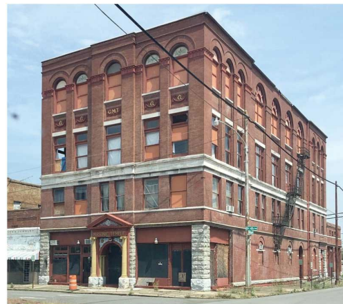
Figure 7. Grand Masonic Temple Exterior
