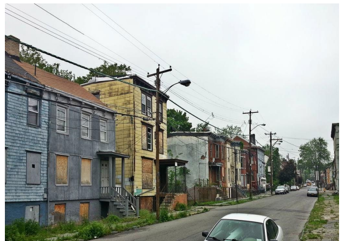
Figure 26. Poor Quality Housing in Newburgh
