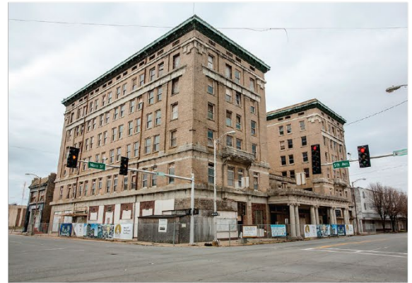
Figure 12. Hotel Pines Exterior
