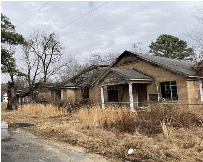
Figure 3. Abandoned home in Pine Bluff
