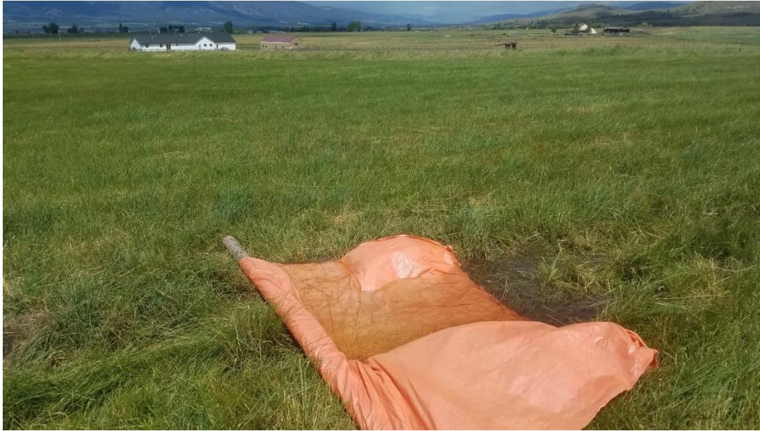
Figure 5: Wild flood or cascade irrigation system in Ravalli County, separate from the one discussed in this thesis. Water flows down a ditch until it reaches the check dam shown above. Here it builds up until it flows over the bank on the downhill side flooding into the field below. Image taken July 18, 2019.
