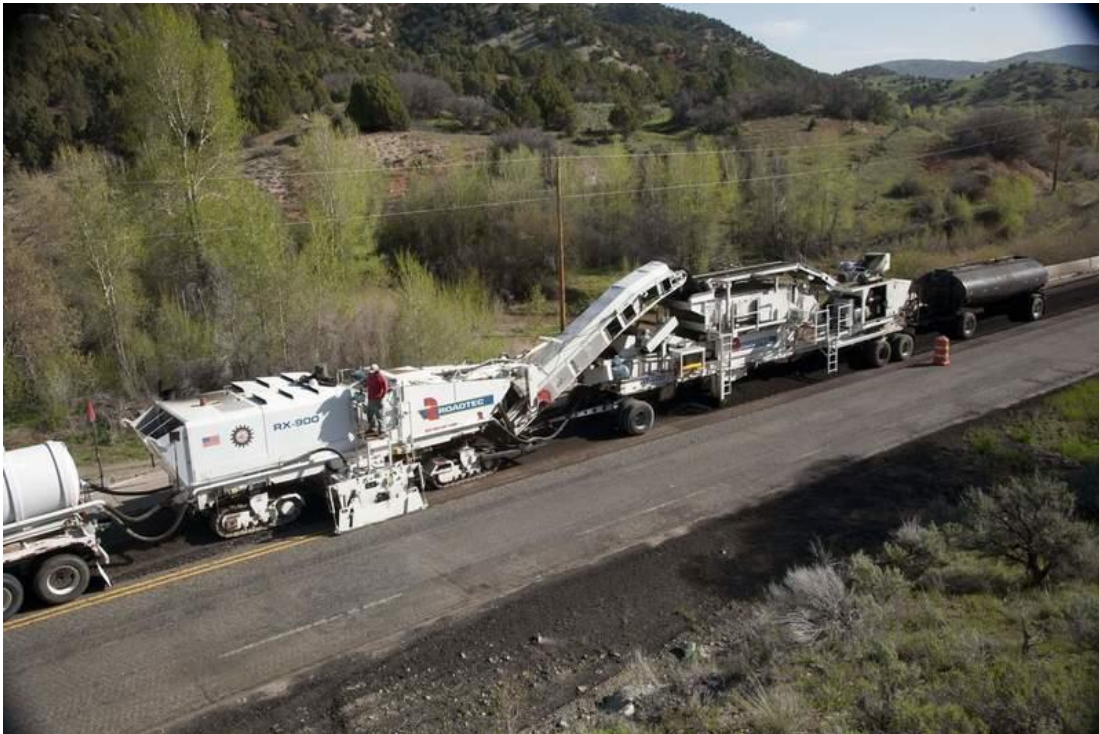
Figure 2: Multi-Unit CIR Train Process (2)
