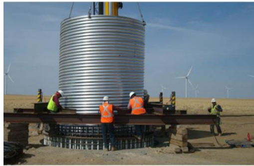
Figure 1-5. Patrick and Henderson foundation (Tensionless Pier Wind Turbine Foundation)
