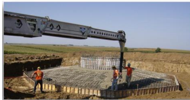
Figure 1-6. Square pad and pier foundation [1] (National Renewable Energy Laboratory, 2001) [2] (Schaefer, 2011)
