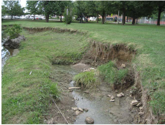
Fig. 6. Picture of southern reach of College Branch Creek showing significant soil erosion.
