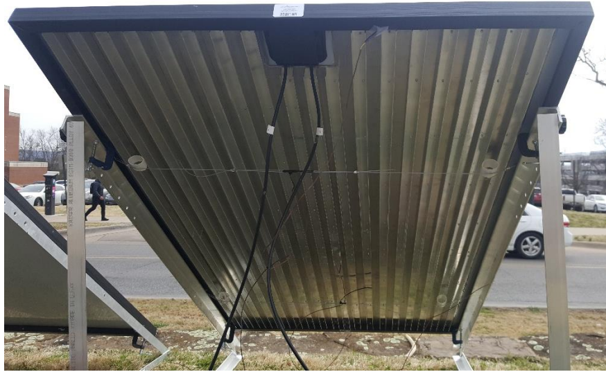
Figure 14. In-House Constructed Fins
