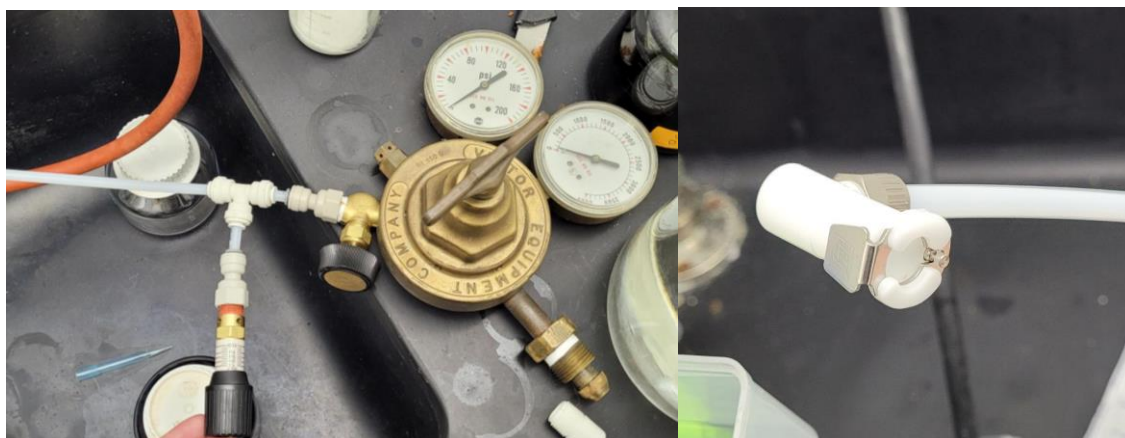
Figure 6. The piping to the gas tank's pressure gauge assembly and ultrafiltration flow cell quick connect
