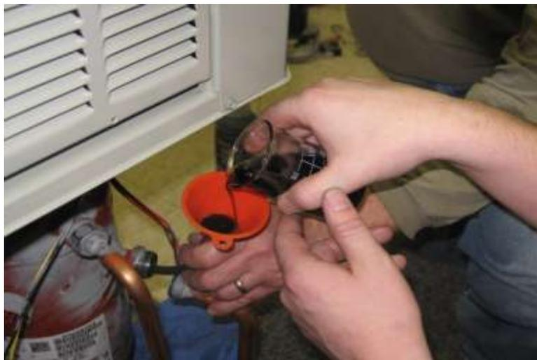
**Figure 2. Pouring CNT/oil mixture into the scroll compressor by way of funnel and tube.**
