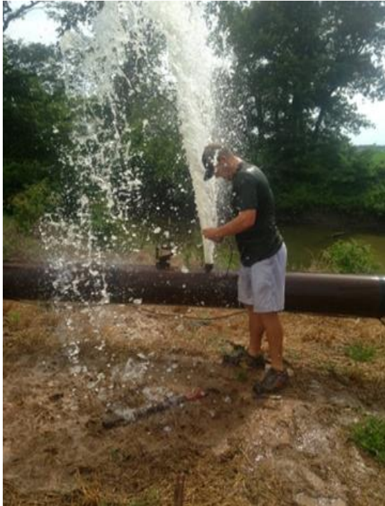
Figure 7. Servicing a Jammed Pump Monitor Flow Meter to Remove Surface Water Debris. Note. Used With Permission from Photographer Colt Oade.
