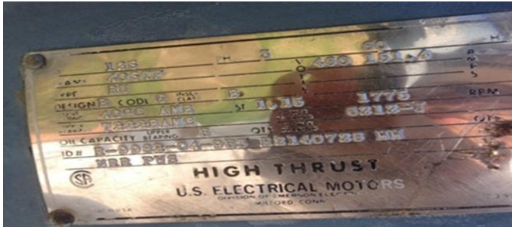
Figure 5. Nameplate from 60 HP (45 kW) Electric Irrigation Motor.
