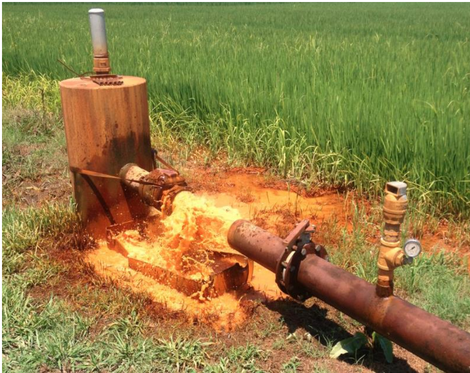
Figure 17. Example of Poor Irrigation Capacity in Prairie County, AR due to Critical Alluvial Aquifer Depletion. The Bright Orange Color of the Water is Due to its High Iron Content.
