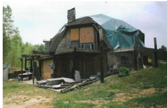
Figure 2.12: A dome house hit by an EF5 tornado in West Jefferson County 1998 (AGE dome)
