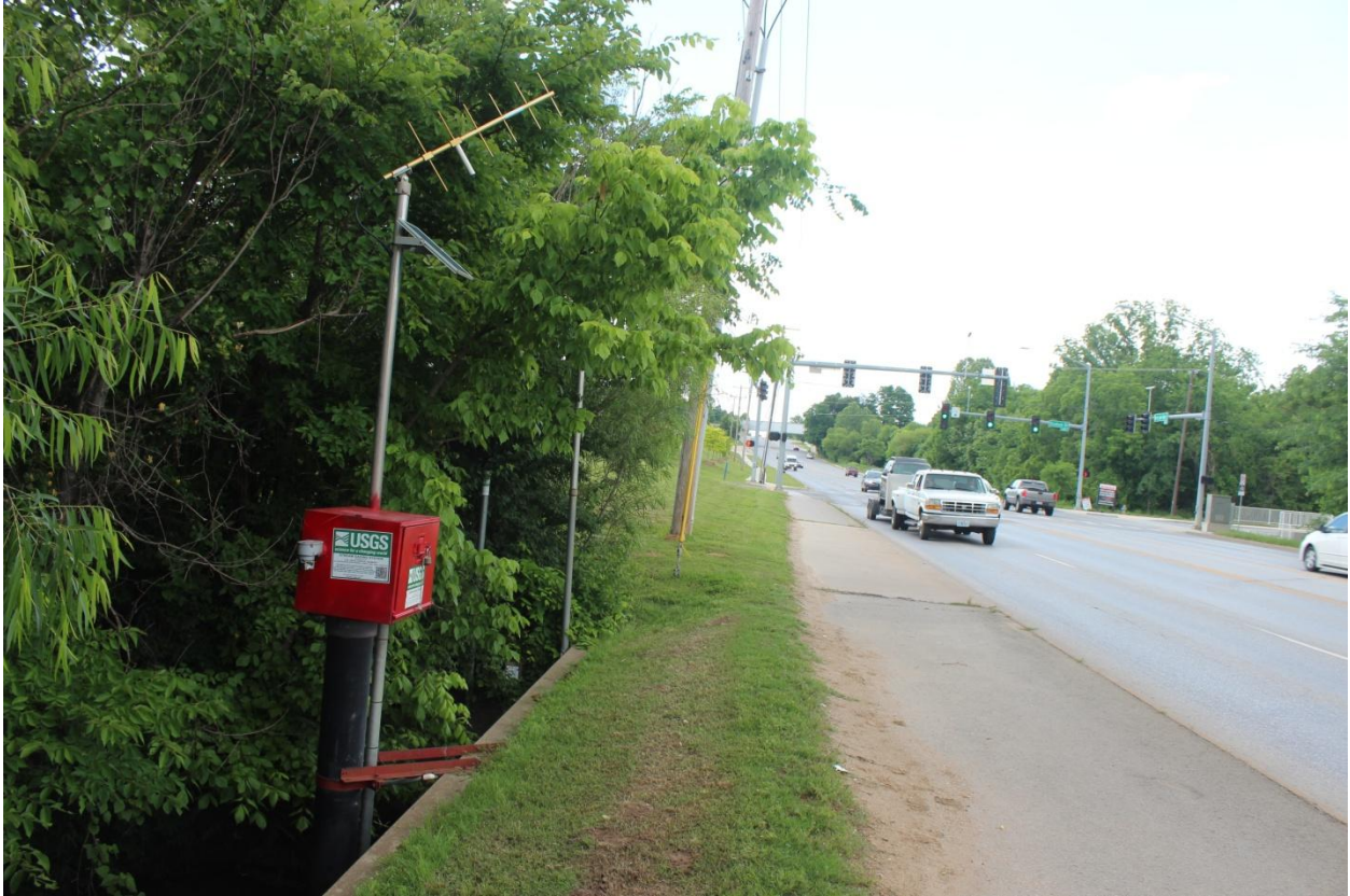
Figure 3.7. USGS Gaging Station (07048480) “College Branch at MLK Blvd at Fayetteville, AR” located where Mullins Creek runs under Martin Luther King, Jr. Boulevard (road to the right of the photo). Mullins Creek is flowing from left to right under the road in this photograph. (Unless otherwise noted, all photographs in this document were taken by the author.)
