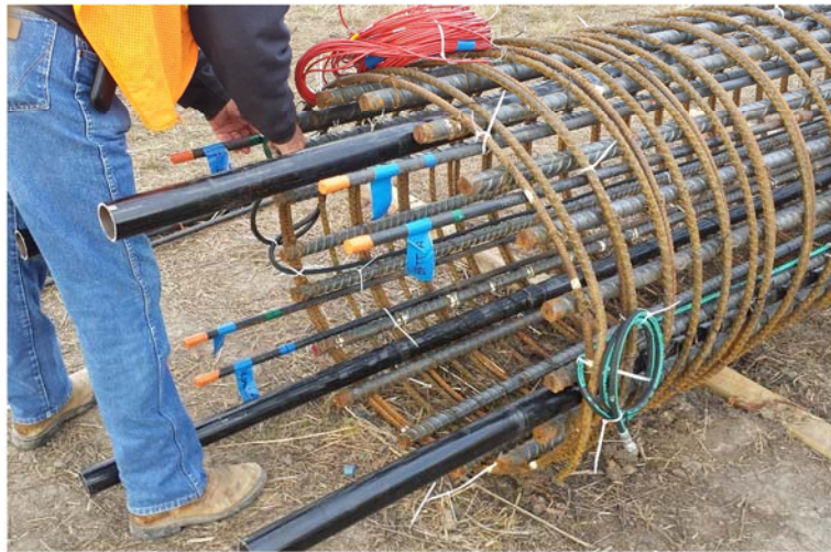
Figure 6.23. Schematic of (a) top-down view of test shaft T-4S, and (b) photograph of instrumented assembly.
