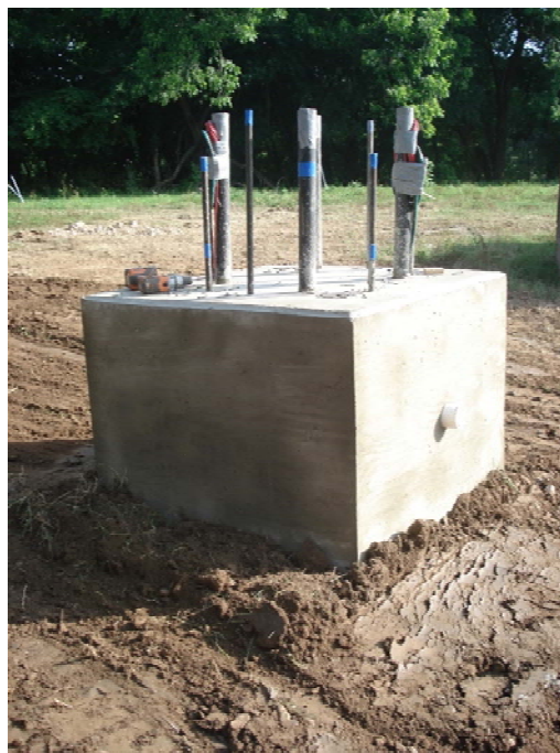
Figure 5.15. Photographs of Test Shaft SS-W4 (a) rebar cage, and (b) finished construction.
