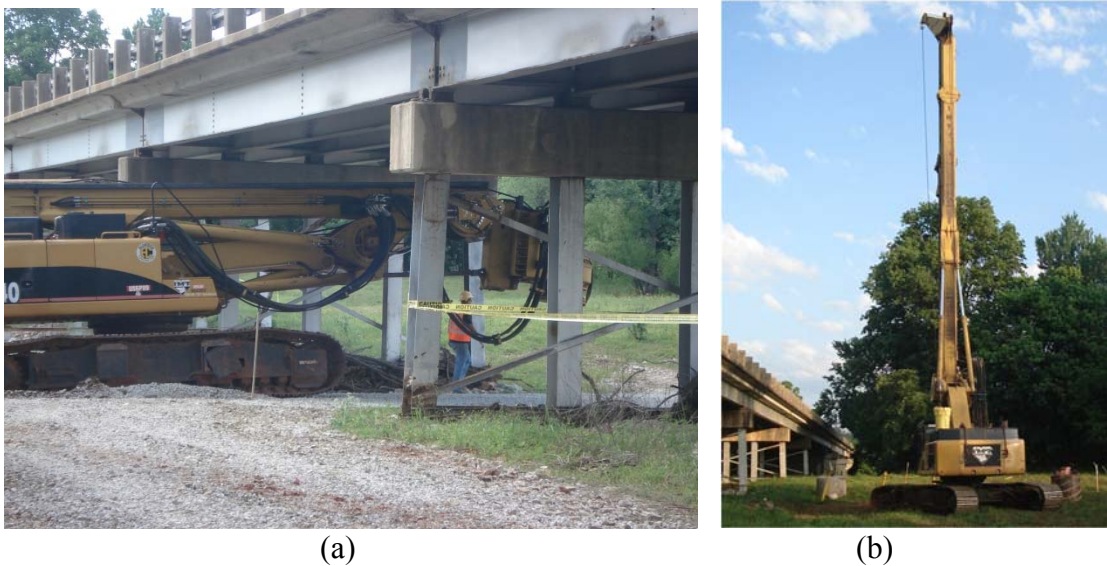
Figure 5.8. Photograph of Caterpillar AF 240 drill rig (a) mobilizing at the Siloam Springs site, and (b) in full operation at the Siloam Springs Site.
