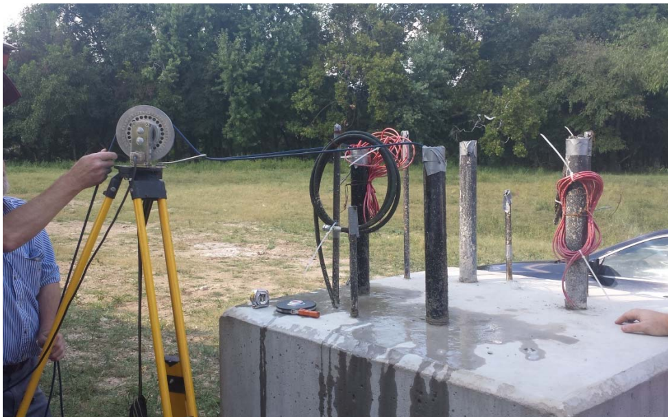
Figure 5.26. Photograph of CSL testing performed on Test Shaft SS-E4.
