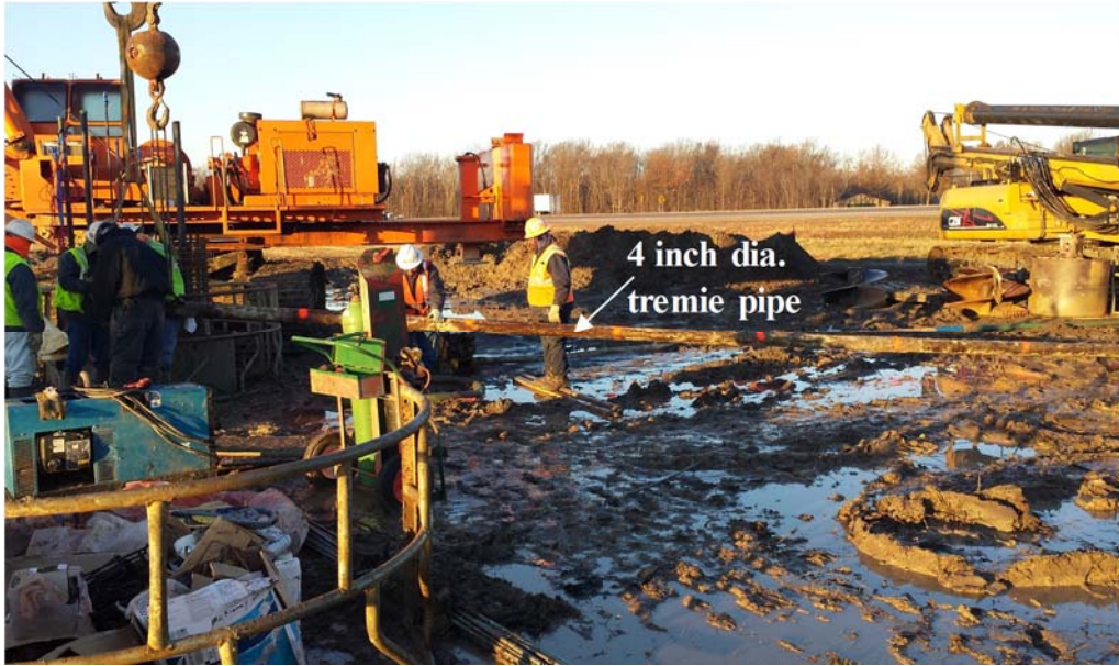
Figure 6.14. Photograph of installation of the four-inch inner diameter tremie pipe for test shaft T-6C.
