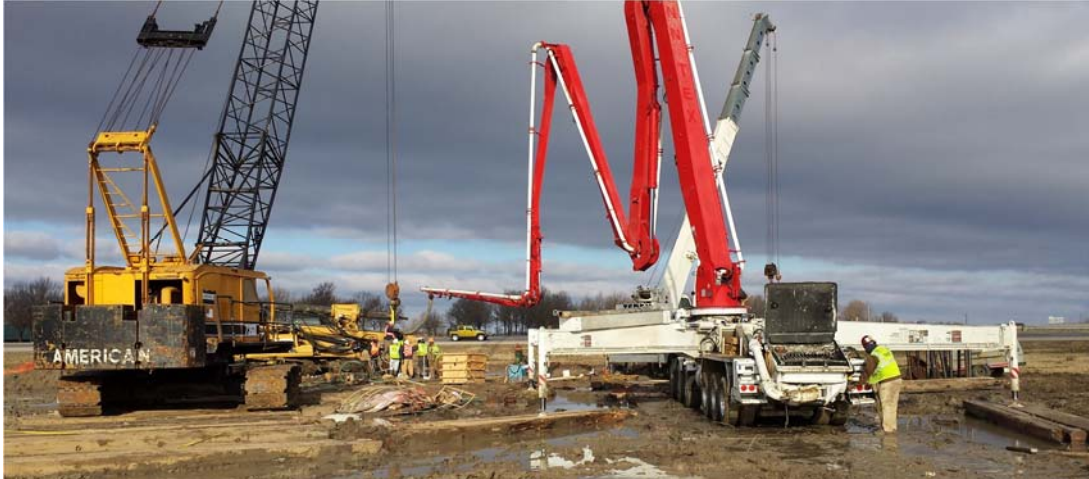
Figure 6.13. Photograph of the Putzmeister 52M pump truck at the Turrell Arkansas Test Site.
