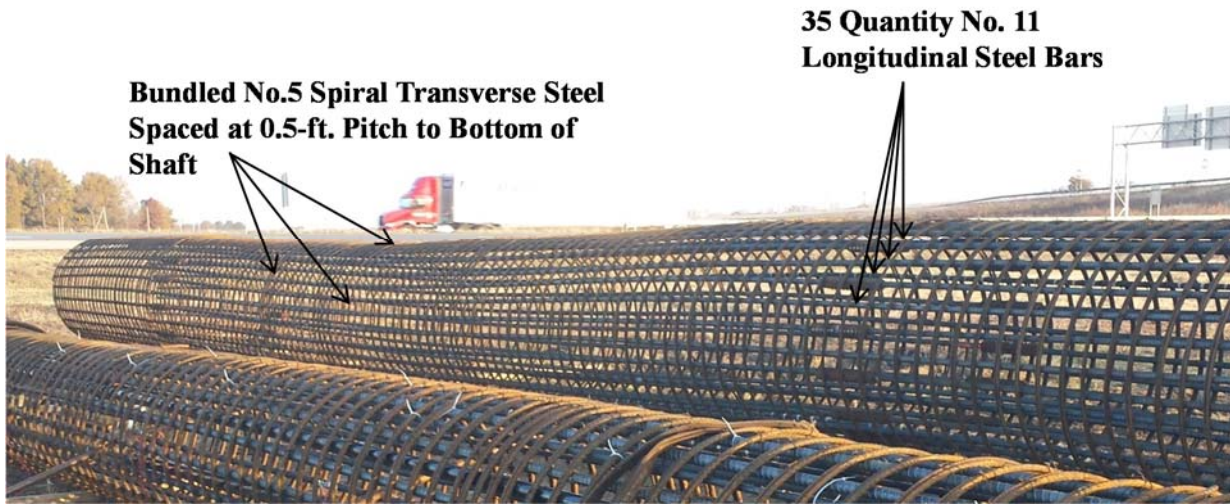
Figure 6.8. Photograph of a side view of the six-foot diameter shaft reinforcement cage.
