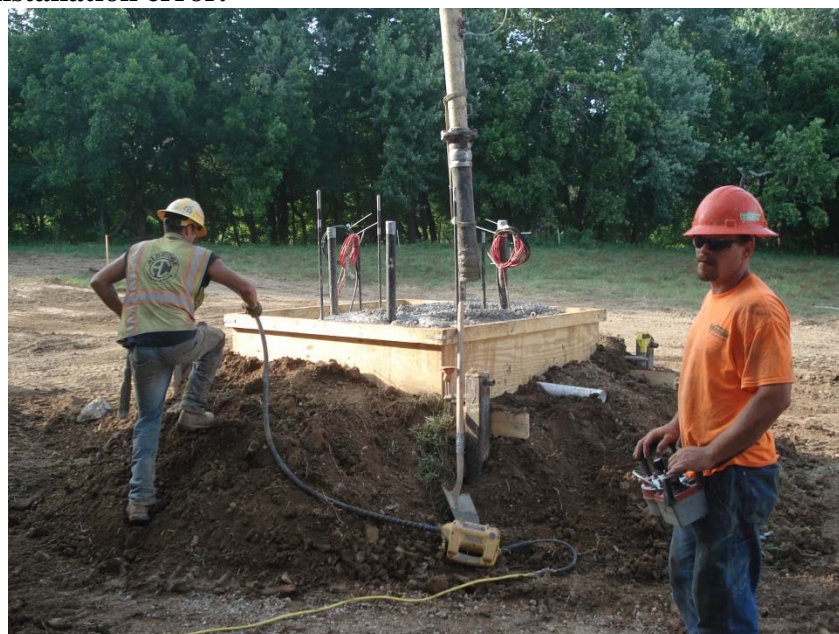
Figure 5.18. Photograph of Test Shaft SS-C6 four-foot reveal construction.
