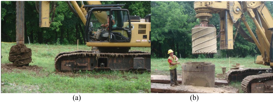
Figure 5.12. Photographs of Caterpillar AF-240 drill rig utilized to excavate Test Shaft SS-W4 with (a) a flight auger, and (b) a rock core barrel.
