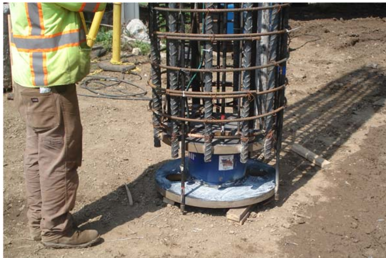
Figure 5.13. Photograph of installed O-Cell on bottom of SS-W4 reinforcement cage.
