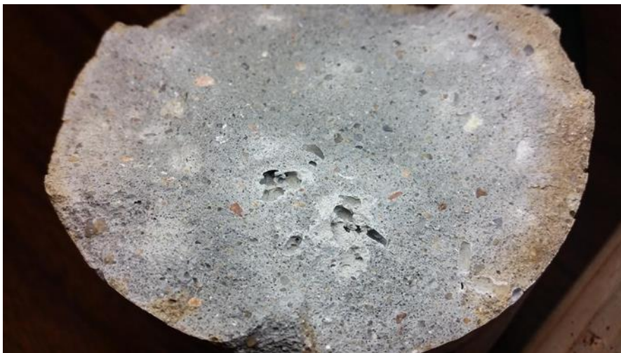
Figure 7. Undissolved chemicals in the mortar
