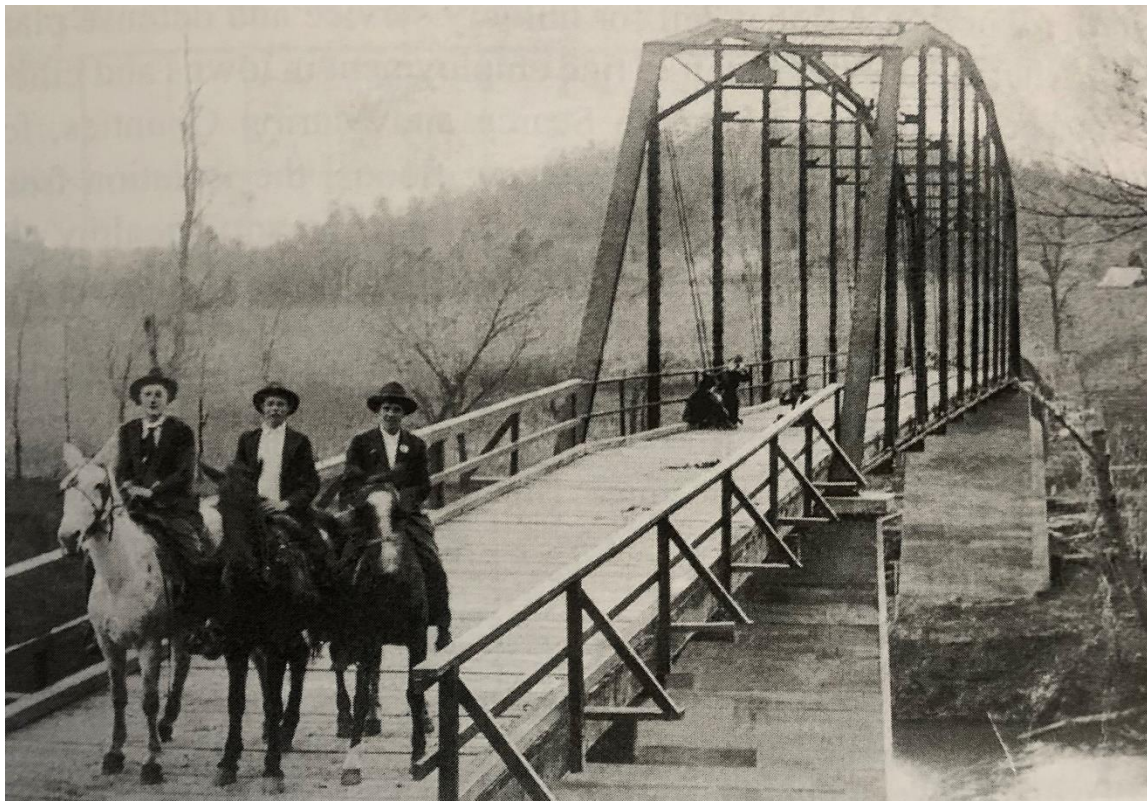
Figure 3.8: The second bridge to span the Buffalo River, pictured above, was built at Carver and completed around 1916 (Ken Smith, 2018, p. 101).
