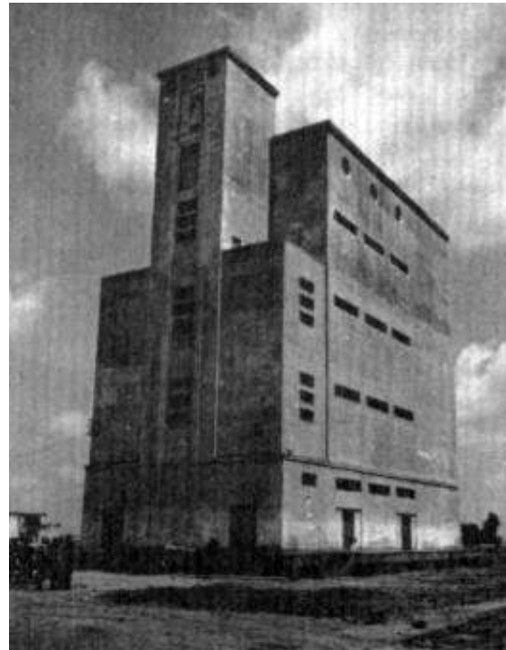
Figure 7.5: The five-story silo building of reinforced concrete construction. The structures with reinforced concrete walls withstood the earthquake forces (Minami, 1965).
