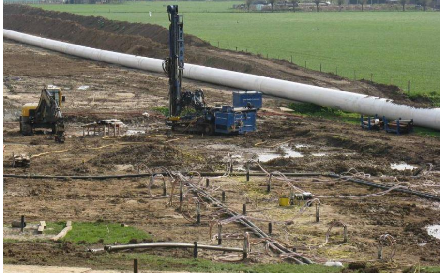
Figure 2.4.1.3 The field where borehole stability was performed (van Paassen, 2011).
