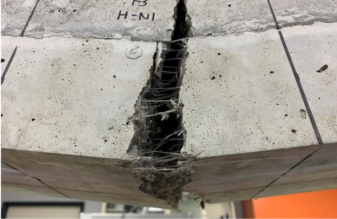
Figure 33. Fiber 3 hybrid beam at end of test.
