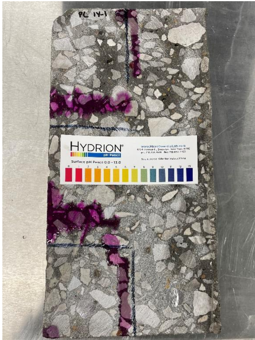
Figure 15. Carbonation test for PC 1y-1
