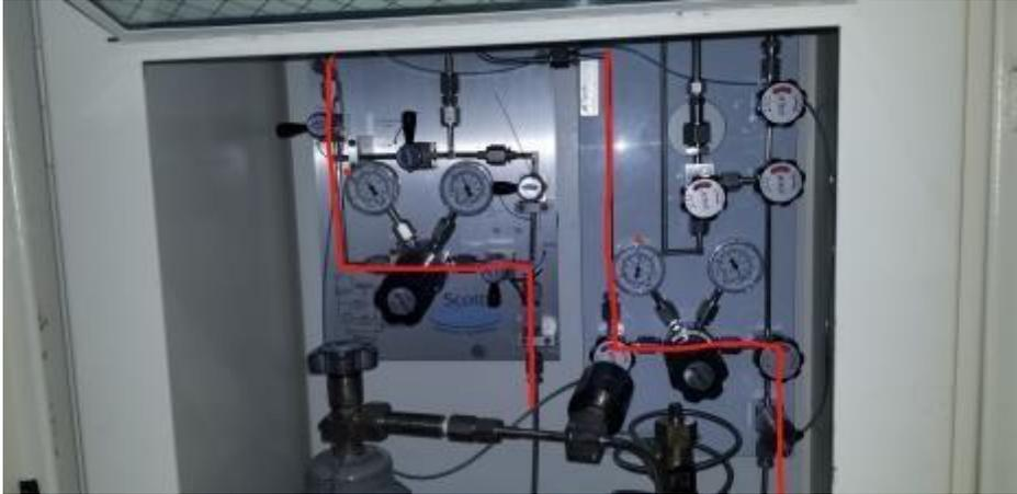
1 - Image illustrates the Cl<sub>2</sub> and BCl<sub>3</sub> gas lines near cylinders. CW turns to close the cylinder.
