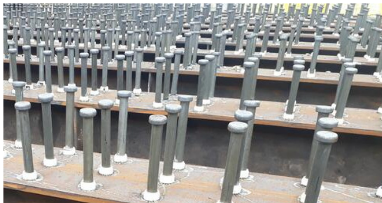
Figure 1 - Shear studs on a composite bridge prior to concrete pour
