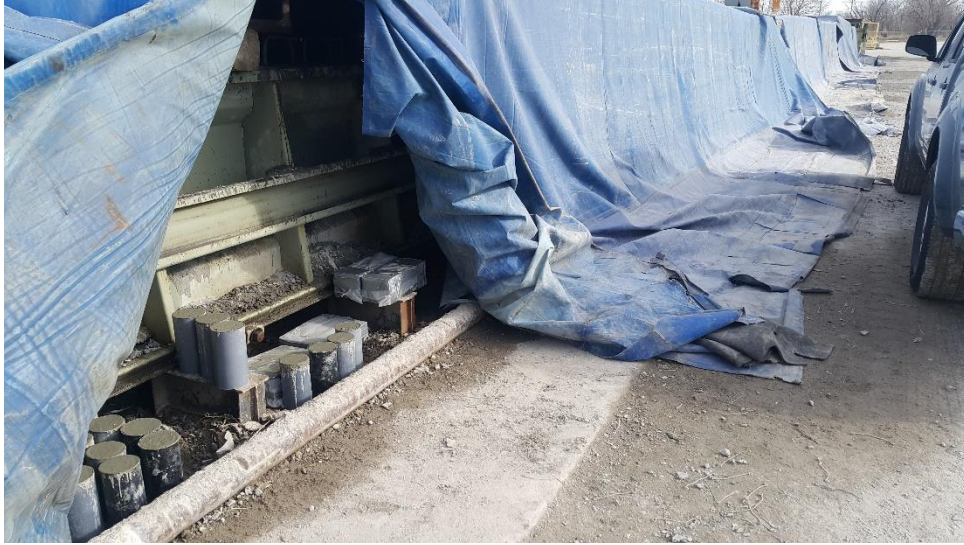
Figure 2. Concrete cylinders placed beside the girders forms
